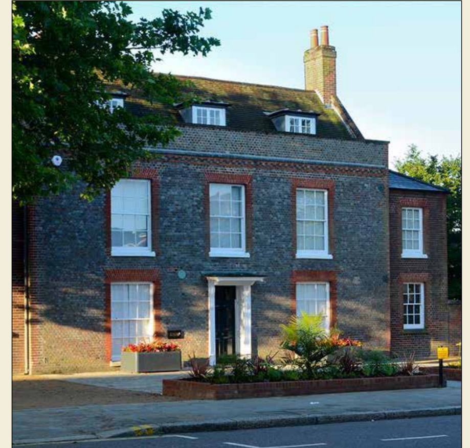
03 - West Street/Westbury Manor
